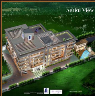
The Marquis (Residential, Ongoing) Whitefield
